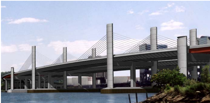
The New Pearl Harbor Memorial Bridge in New Haven, CT
